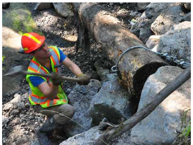
Cabbling a log to protect creek bank.
